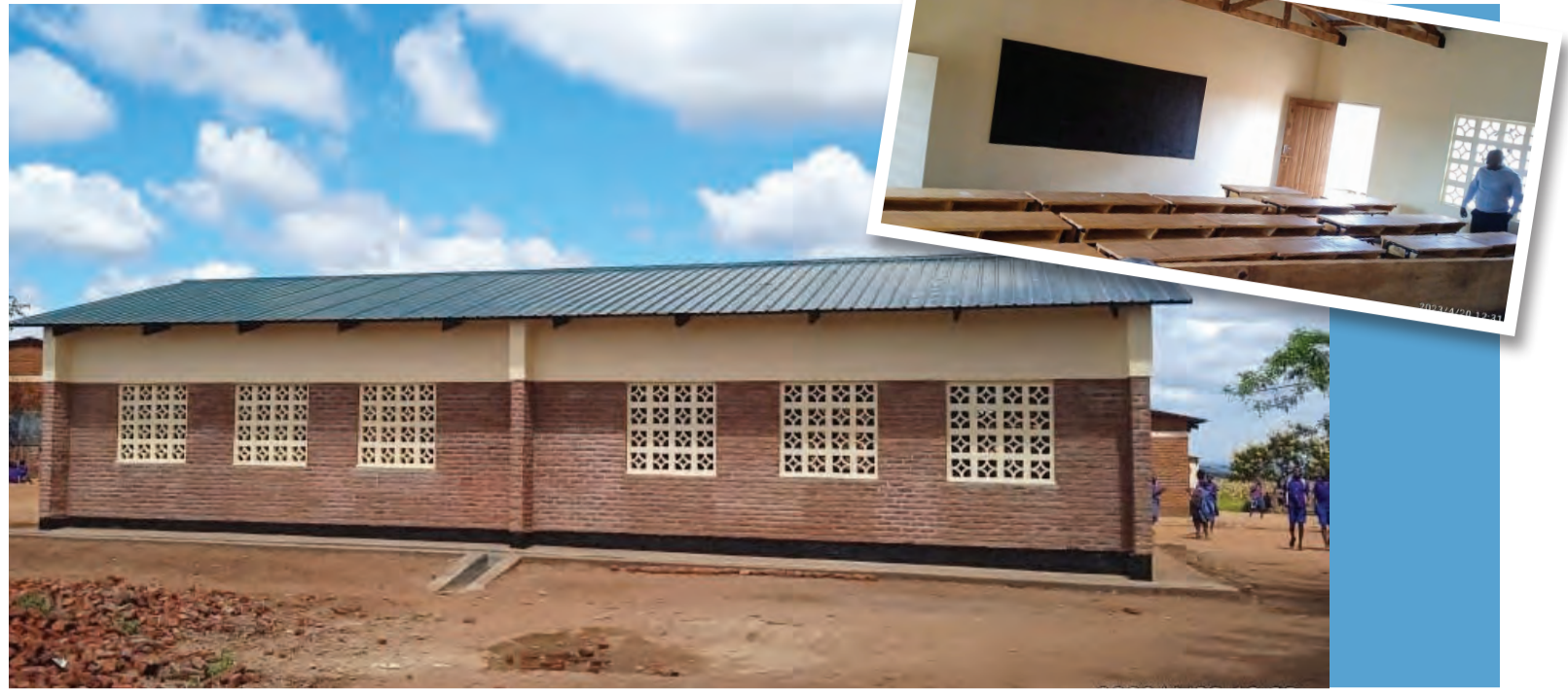
The classroom block during construction Photos: Innocent Mofolo
